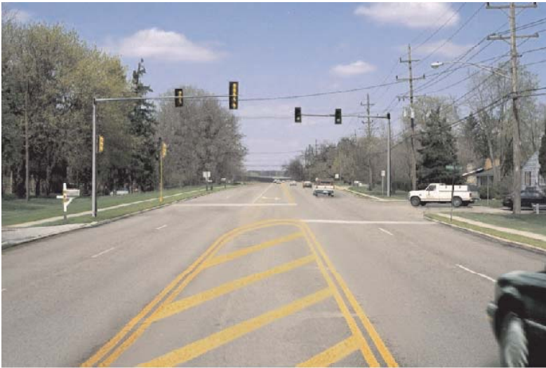
Figure A: IDOT's original plan for Lombard. Five-lane road design with sidewalks 3 feet or less from the curb.
